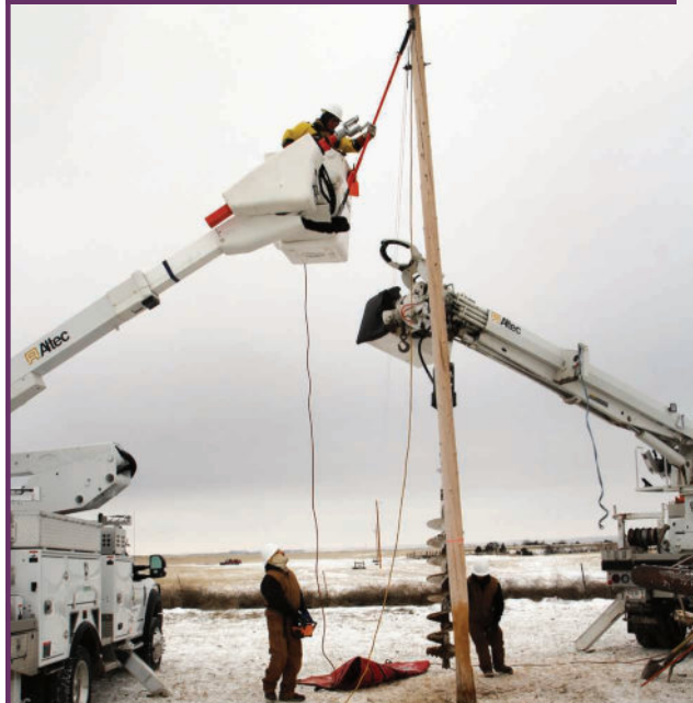
Black Hills Electric's Crew Foreman Dean Whitney and journeymen linemen Beau Bradeen, Ken Parker and Corey Scott replace poles near Red Shirt, S.D.
