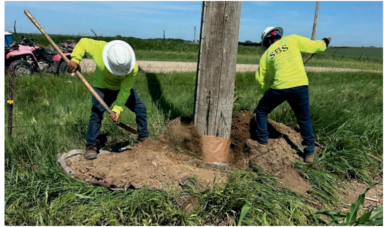
Photo courtesy SBS Inspections, Inc.
