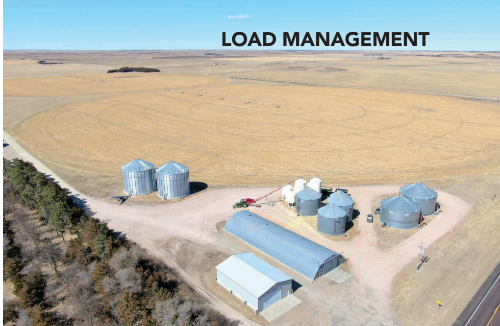
All of the roughly 200 irrigation pivots at Danielski Farms are under Cherry-Todd Electric’s load management program.
