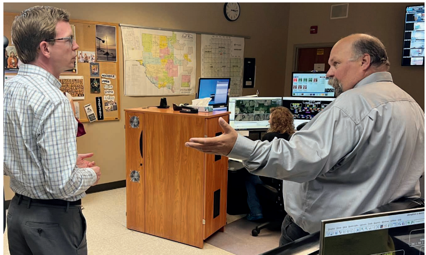
During a visit to Sioux Valley Energy's Colman office in late June, Rep. Dusty Johnson, left, listens as Sioux Valley Energy Vice President of Engineering and Operations Ted Smith, right, explains how the Co op's dispatch center works. Dispatcher Eliza B. is seated at one of the center's work stations.
