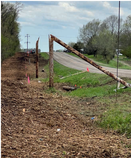
Left: Line leading into the Oldham substation in Kingsbury County was damaged. Above: A crew splices a line near Hills, Minn. Below left and below: Damage to a stretch of line in Brookings County required removing a half mile of tree debris and broken poles before repairs could be made.
